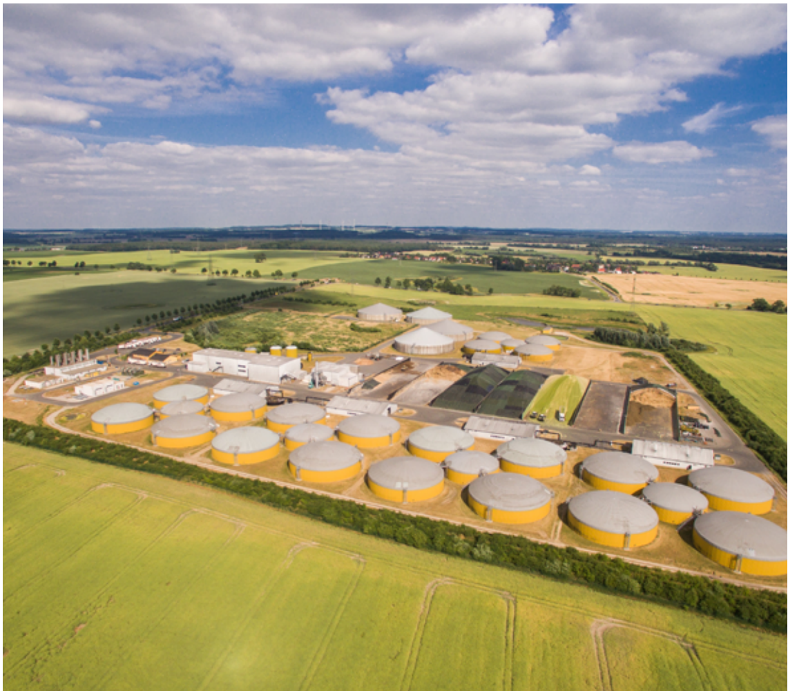
Large biogas plant in Germany.
